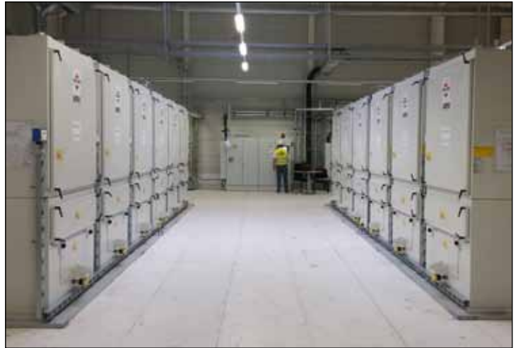
Central separation system with twelve AERO® modules, size 3 Nominal air flow 140 000 m 3 /h
