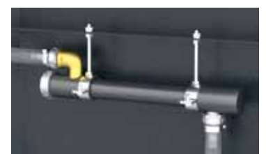
An optional UV-light prevents the propagation of hazardous bacterial growth. Recommended for prolonged use of process water.
